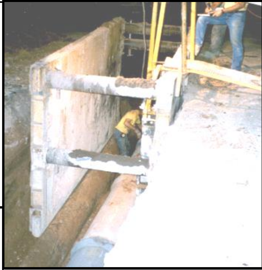
A trench shield
